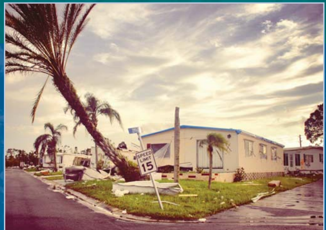
Hurricane damage in Florida illustrated here is a familiar fact of life this year.
